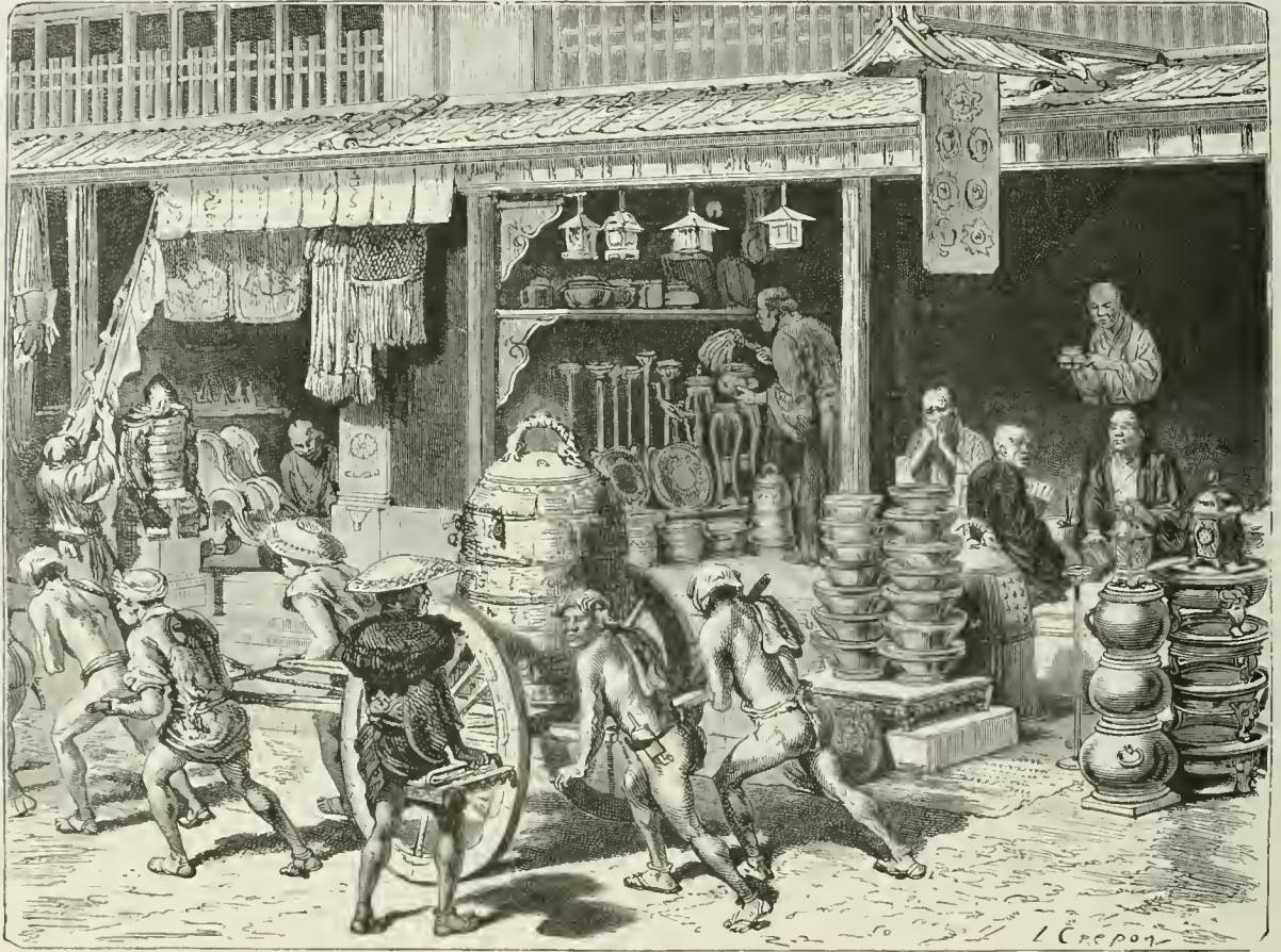
A BRONZE WAREHOUSE AT YEDDO.
